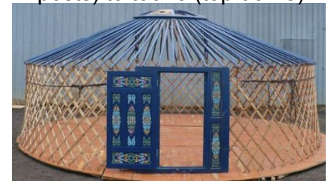
4. Put hun (roof rafters). Adjust tension with circular tension rope and make sure the toono is placed symetricaly toward in the circle.
