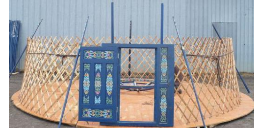
3a. Attach bags (central posts) to toono (top dome)...
