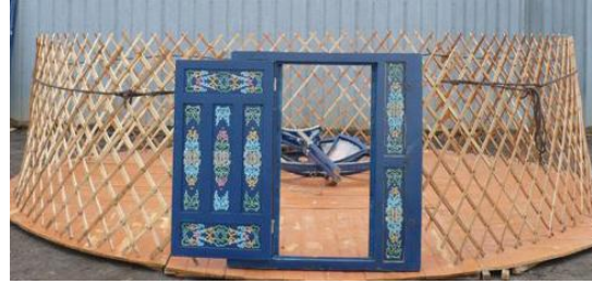
2. connect walls in a circle a add tension rope
