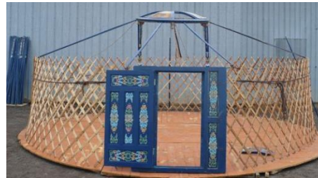
4. Put hun (roof rafters). Adjust tension with circular tension rope and make sure the toono is placed symetricaly toward in the circle.
